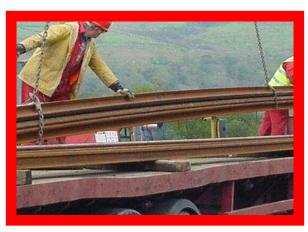
Never lift using chains in contact with the rail
