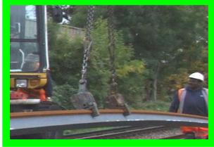
Use correct rail lifting clamps
