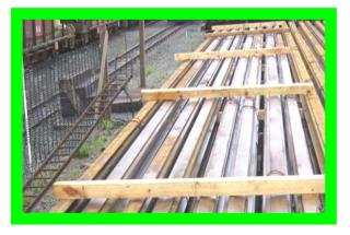
Wooden bearers should be used for stacking to protect the coating sacrificial properties
