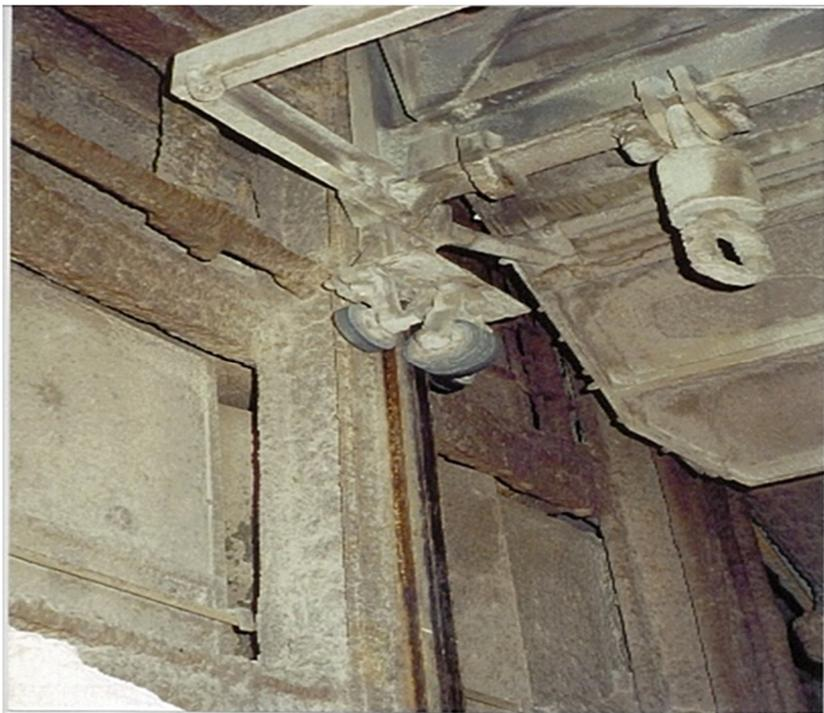
Overall the tophat guide provides a high capacity hoisting system with improved longevity in service compared to other guide systems. More details can be found at: <https://britishsteel.co.uk/what-we-do/special-profiles/mining/>.
